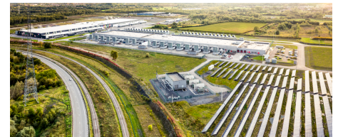
Fluence and Centrica are providing and optimising Google's first zero-emission backup power system for a data centre in Belgium.
